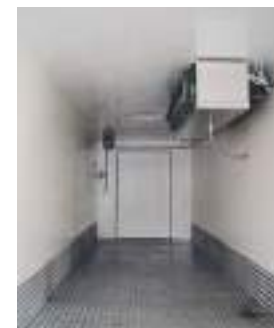
ISO container interior with production room installed above the ice deposit
